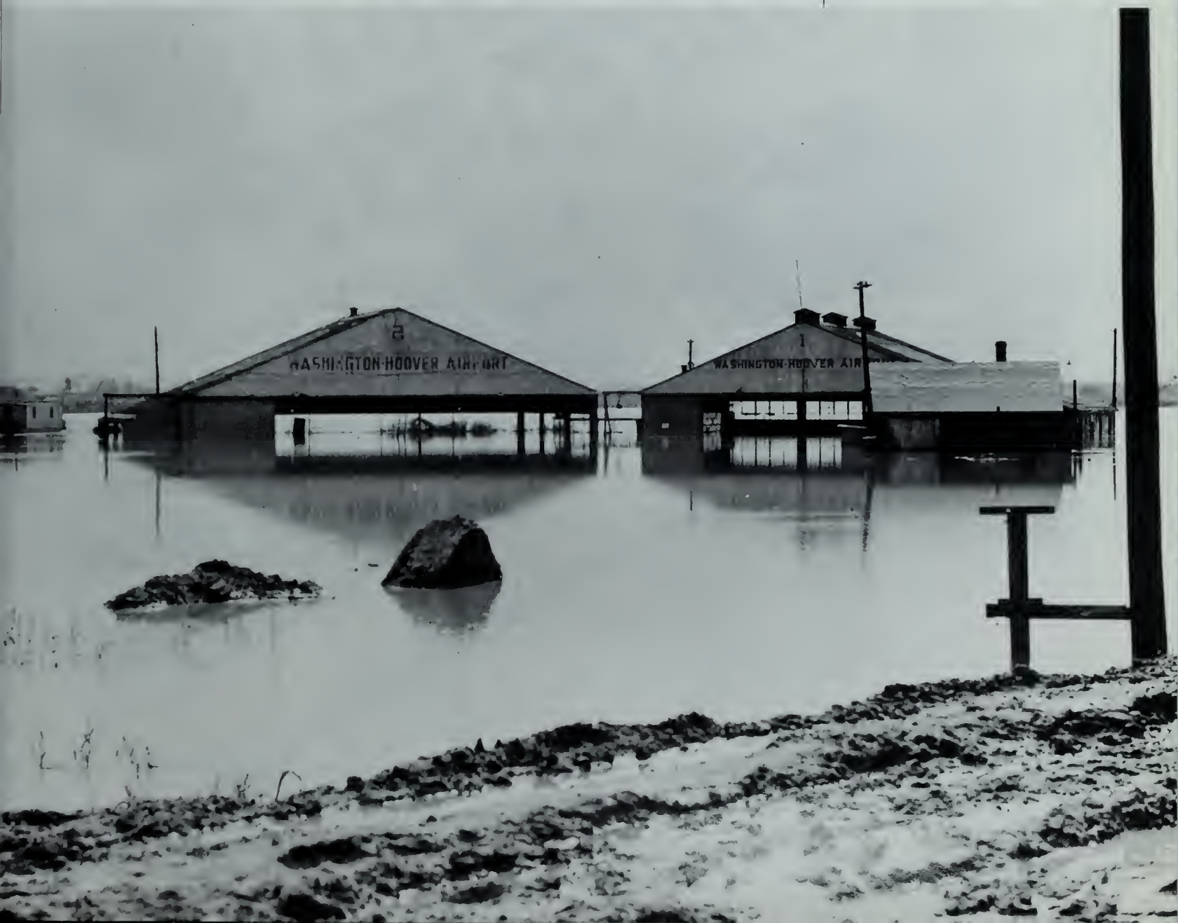
Flooding on Hoover Airport site
